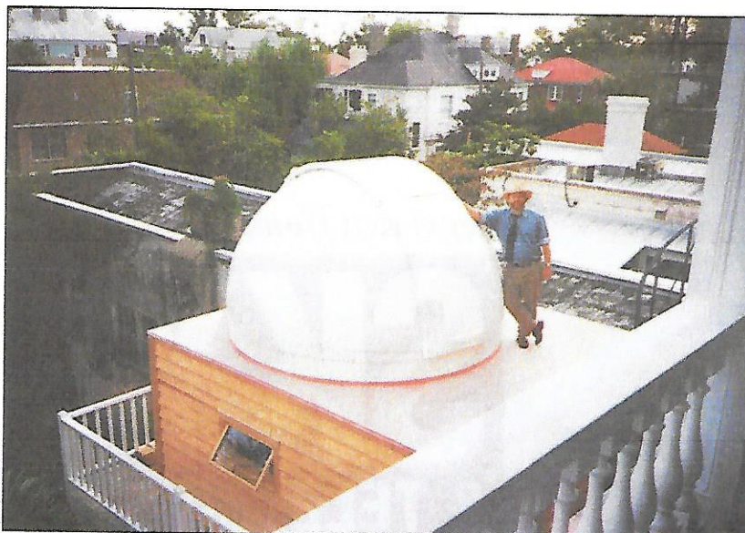
Left: Phillips's observatory was built around his telescope and pier, which are permanently installed on a small deck over his kitchen. Limited space had ruled out earlier designs that called for a roll-off roof or lifting a dome with a crane. All photographs with this article are by the respective authors. Right: Jim Phillips with his 10-foot Home-Dome. The observatory was built and the dome assembled by two carpenters who had no previous experience working on an observatory.
