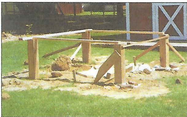
Left: Castle's observatory base is a 12-foot-square deck supported by these four 6-inch-square pressure-treated wooden posts set into concrete. The octagonal, 4-foot-high walls are made of 2-by-4 studs with 2-by-6 lumber forming the top plate upon which the dome's base ring sits. The siding is rough-sawn cedar, and a door is included in the northern wall section. Right: The Home-Dome kit can be shipped in a 750-pound box that the purchaser is responsible for removing from the delivery truck. The crating charge for truck shipment is $250, and transportation costs in the contiguous United States range from about $100 to $250 depending on the distance. The dome can also be picked up from the factory with a $50 charge for packing materials, but even out-of-state owners must then pay a 5 percent Maryland sales tax.
