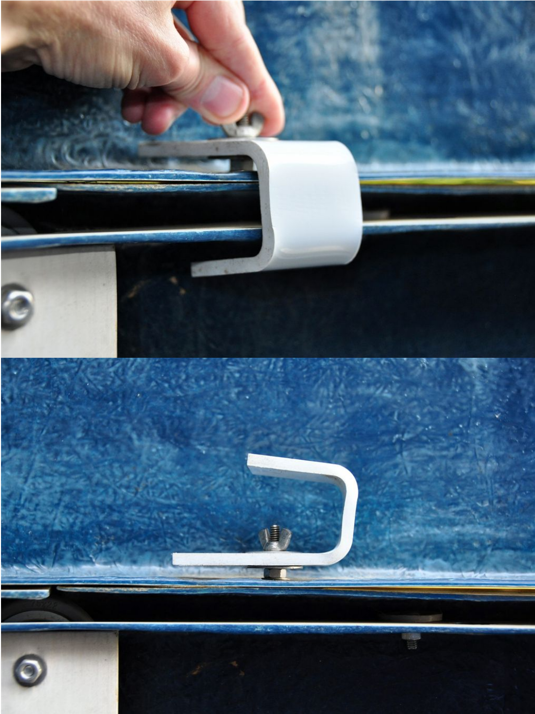
Figure 2: Four dome hold-down clamps are used to secure the dome when not in use. The dome rests on a series of rollers which enable the dome to be rotated easily by hand for viewing in any desired direction. The upper photo shows the clamps in the “hold-down” position and the lower photo shows one of them in the “standby position”. To be able to rotate the dome and use the observatory, the clamps must be in the “standby position”. The hold-down clamps ensure the dome does not lift or shift position in high wind conditions when the observatory is not in use. Always return the hold-down clamps to the “hold-down” position before leaving the observatory.
