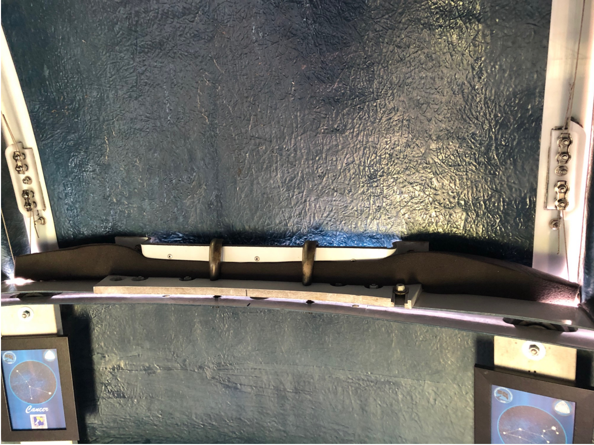
Figure 10: Before fully closing the shutter door, insert the foam cushion shown to prevent entry of birds and insects. Carefully compress the foam under the door as it is closed. Then insert the J-hook bolts as shown in the next Figure.
