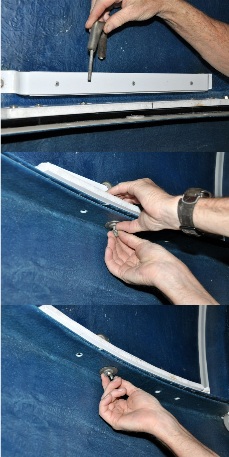
Figure 11: Once the shutter door has been closed, insert the two J-hook bolts over the handle of the door and through the holes in the flange of the dome support ring as shown. Use washers and tighten the wing nut snugly to secure the shutter door.
