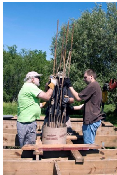
Terry and Eric insert the rebar structure into the tube and orientate it per Rusty's instructions
