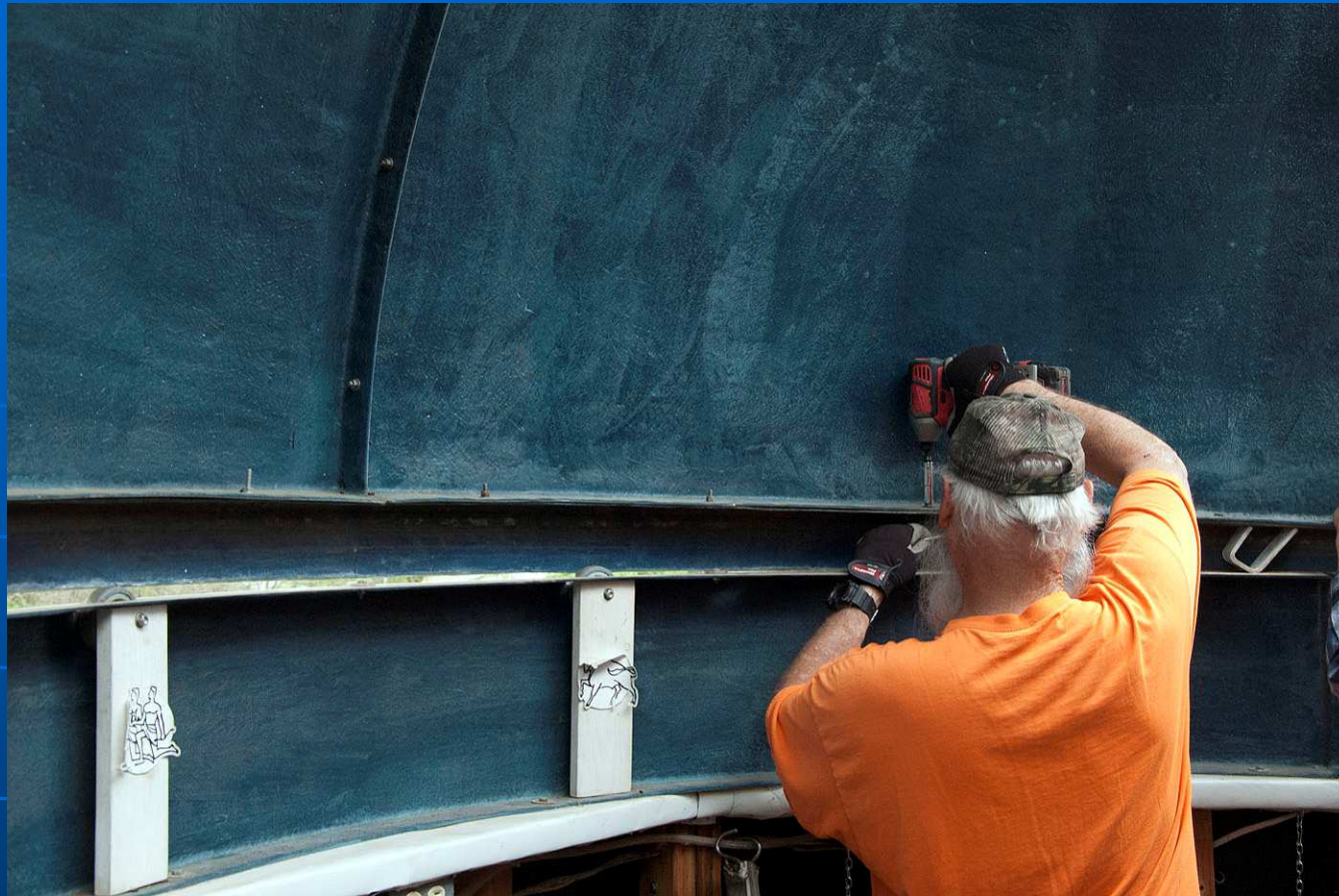
Removing the nuts and bolts inside the dome.
