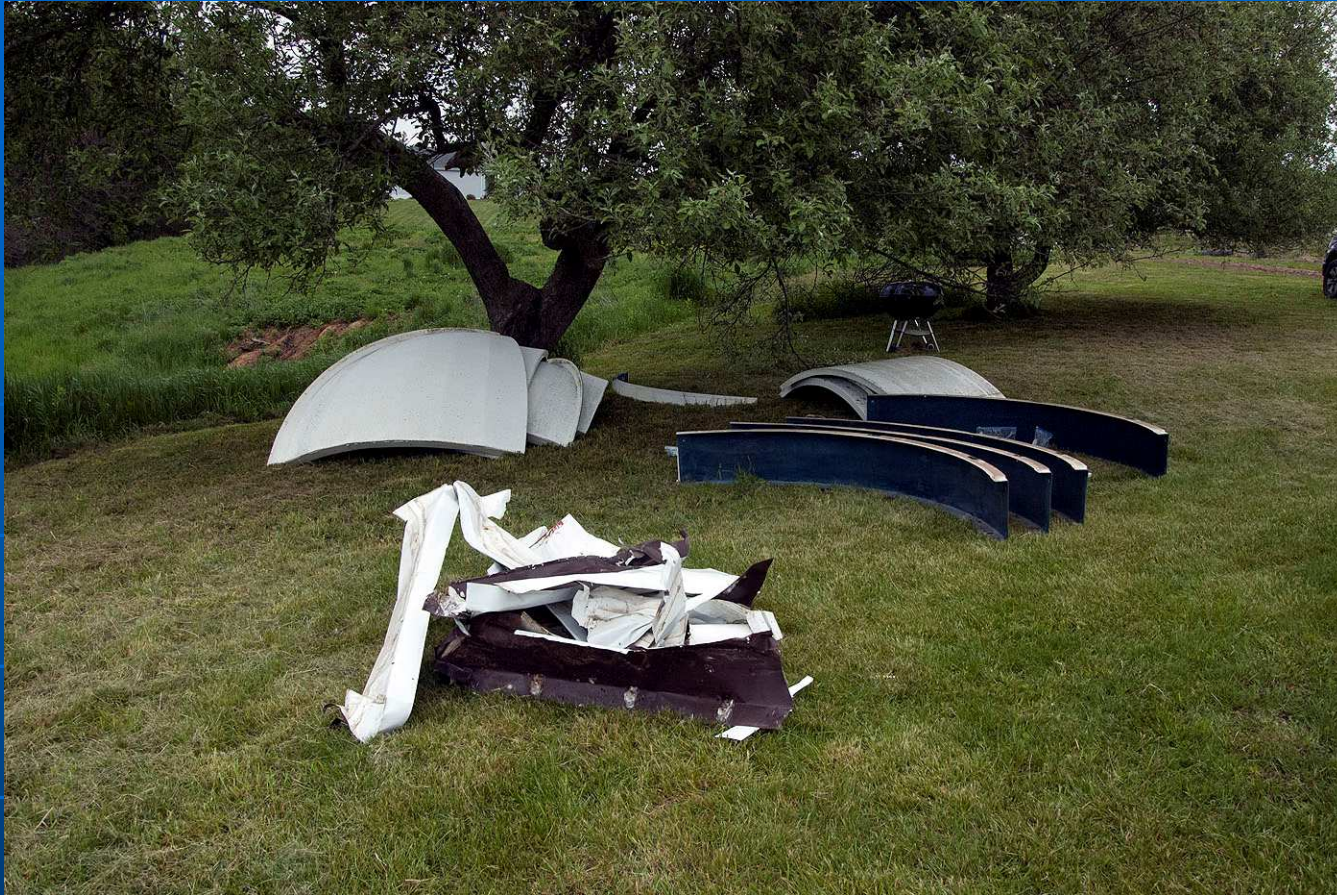
The four dome pieces, the sliding sections, the rolling-sections and the removed aluminum wood frame covers. Ready to move for cleaning.
