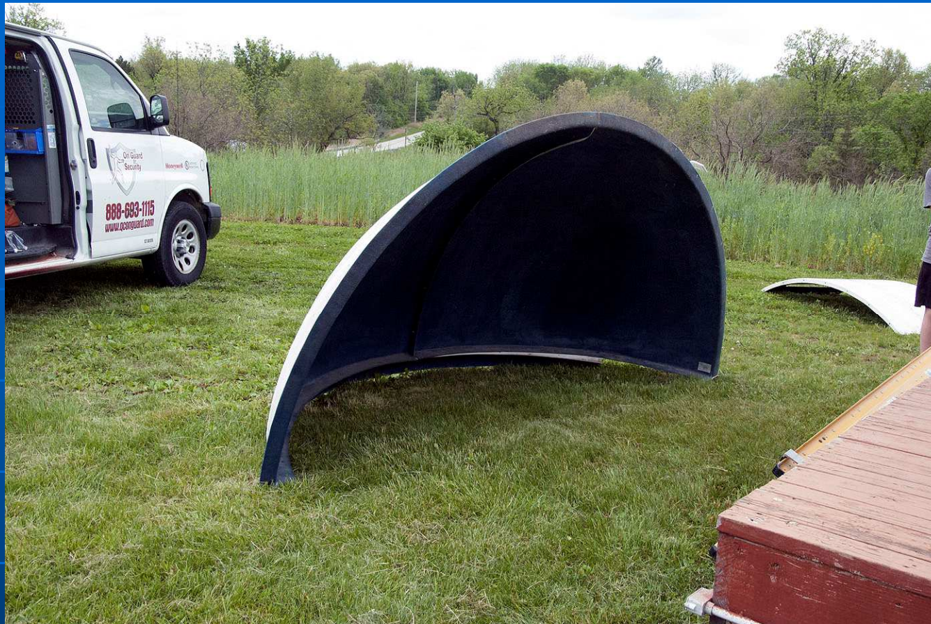
The first two sections removed.
