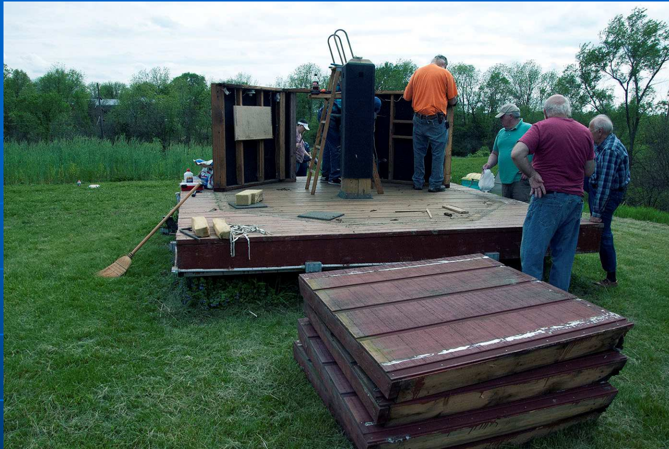
Removing the last three wood frame sections. Five more are stacked in front.
